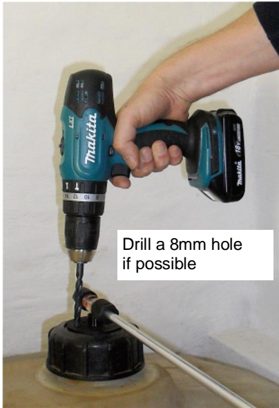
Measuring pipe mounted in tank ventilation
