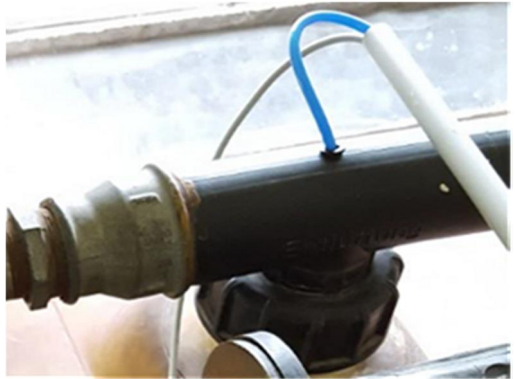
Measuring pipe mounted in tank ventilation
